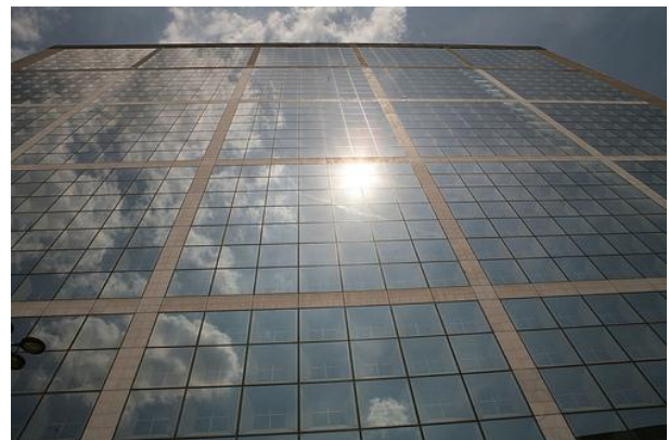
Fig. 1: Not a greenhouse, but offices – thanks to double glazing (photo: Bill Holmes)
